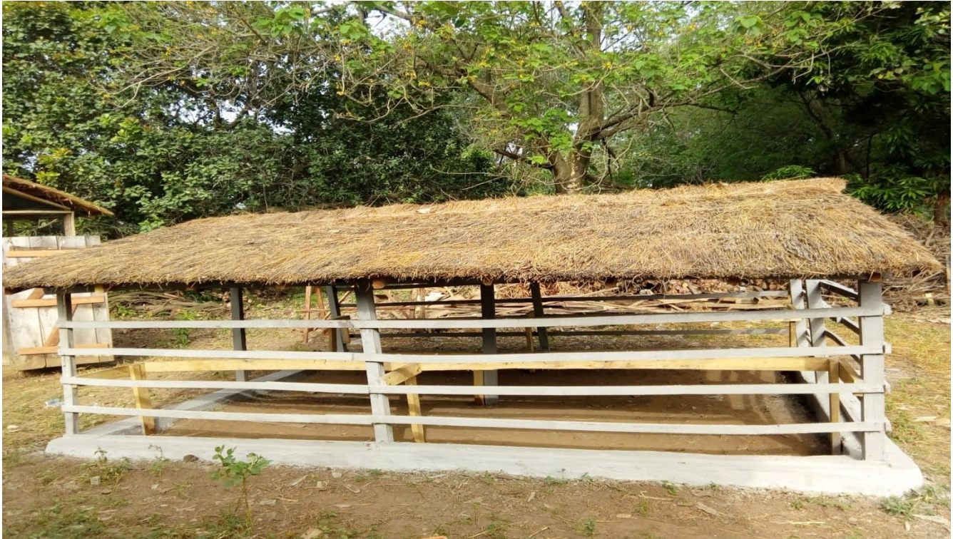
FRESH CASSAVA STORAGE STRUCTURE
