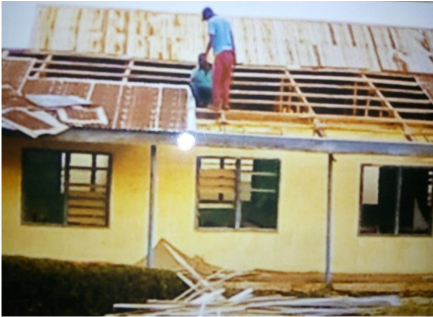
(c) Demolishing of Hall11
