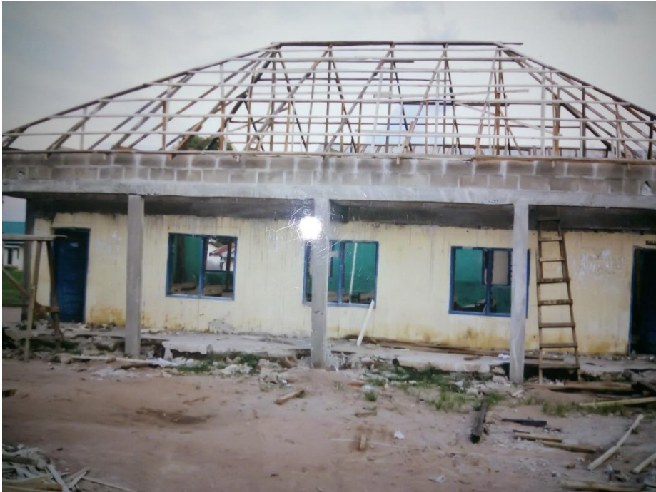
(e) Renovation of Hall 11 in progress
