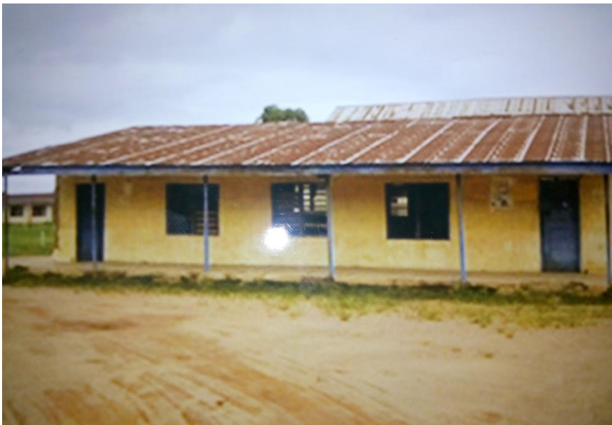
(b) Hall11 before renovation
